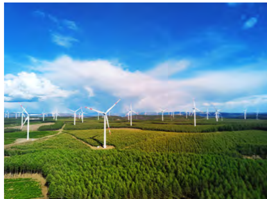
Haizhuang wind turbines in the Saihanba forest farm
